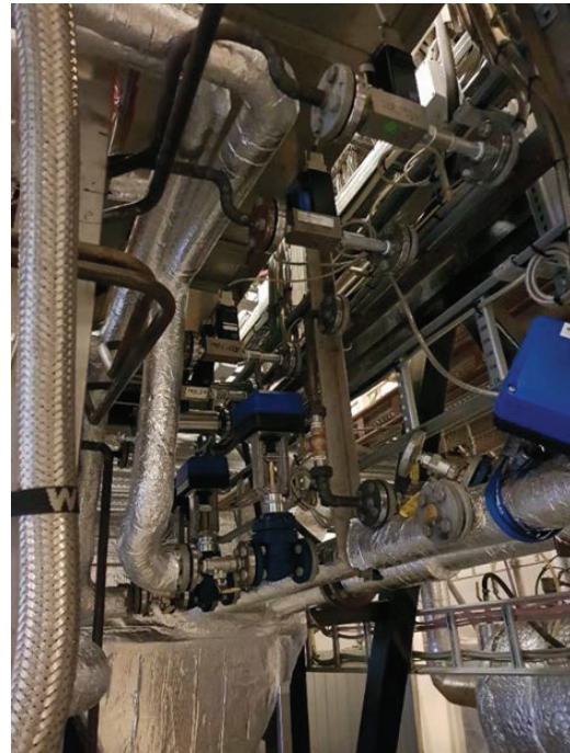
Figure A-2: Thermal mass flow controllers for loop seal and lifter fluidisation
